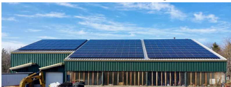
The St. George Transfer Station bedecked with solar panels . . .
