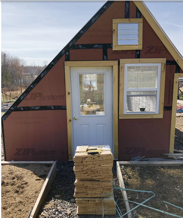
Waiting to be shingle clad - W.McI
