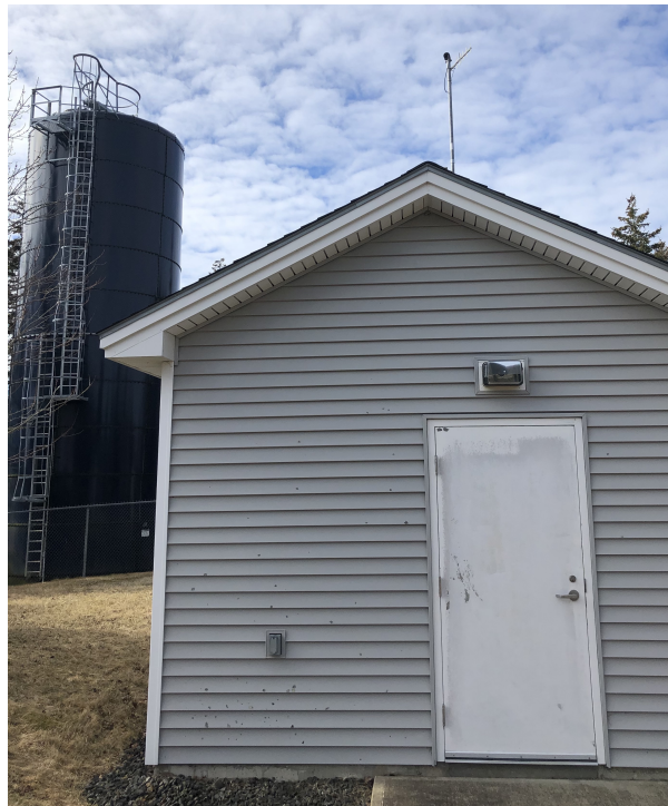
The little booster station that could . . .
